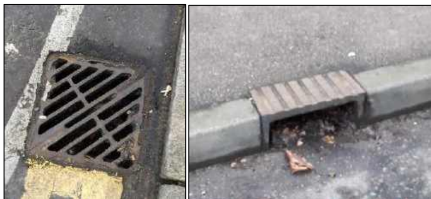
Figure 3-10 Type S and Kerb gullies
